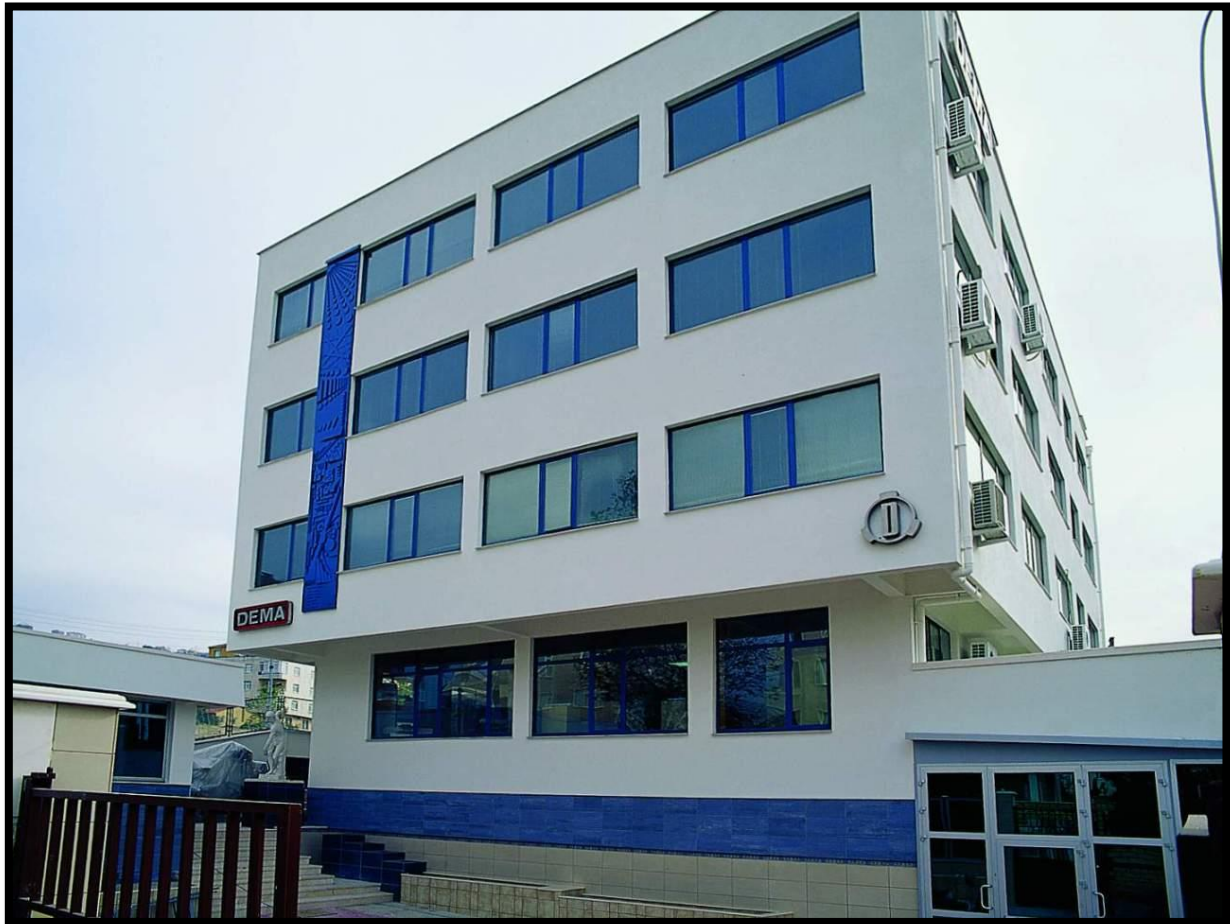
DEMA Role San. ve Tic. A. S. Plant at Istanbul, Turkey.
